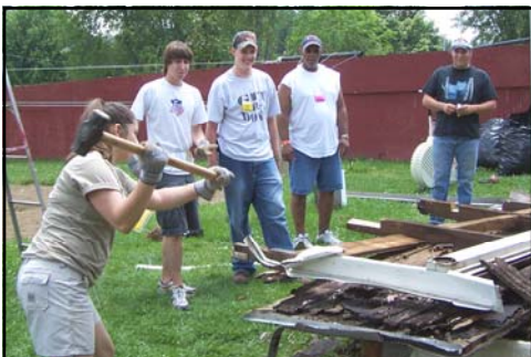
Work team removing porch to do repairs on the house.
